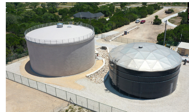
Comal County, TX – This 750,000-gallon water storage tank was completed at a cost of $2.2 million. It is one of 13 water storage projects completed, under construction, or in design.
